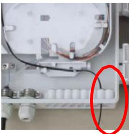
8. Installed the connectors from the drop cables into the bulkhead connector of drop cable
