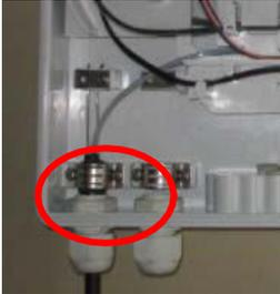
2. Connect the cable with the splitter input cable by fusion splicing or mechanical splicing.
